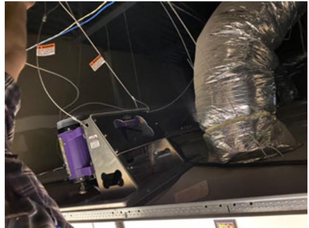
Safety lanyards **MUST** be attached to a load bearing point above the drop ceiling that is capable of supporting 400 lb. Failure to secure the ceiling mount to a proper load bearing point could result in serious injury.
